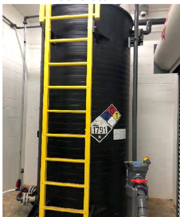
Chlorine Storage Tank
