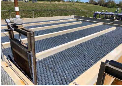
Chlorine Contact Tank
