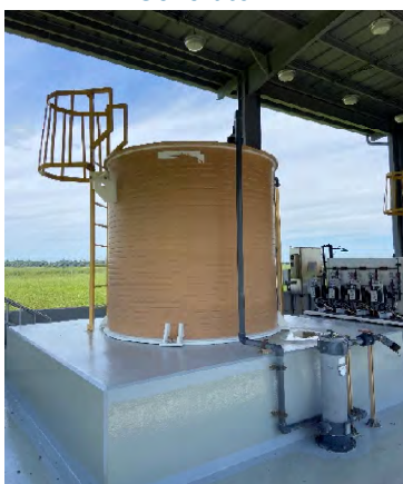
Sodium Hypochlorite Tanks
