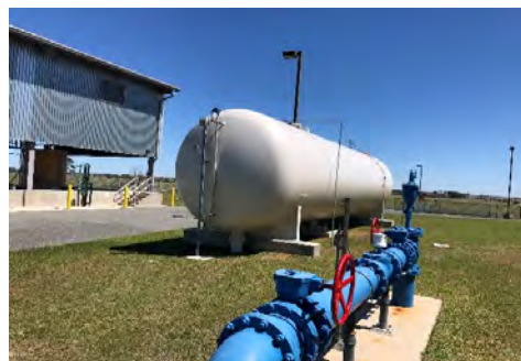
Hydropneumatic Tank
