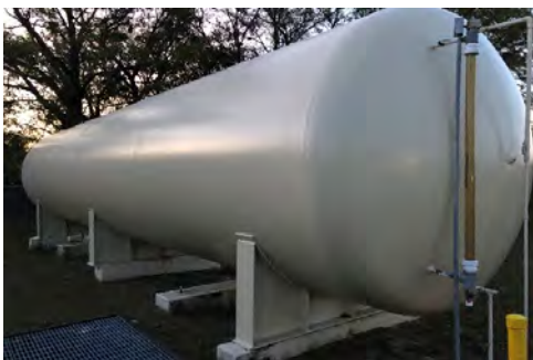
Hydropneumatic Tank
